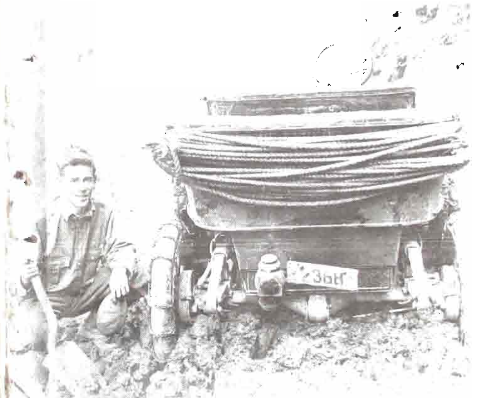
Highway near Newport, 1912
